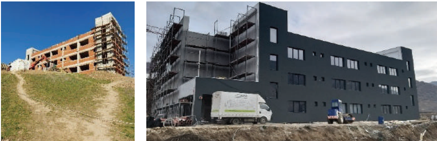
Photos from the construction process (private photographs)
